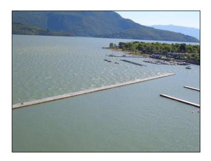
Domaso 2 is the extension of the breakwater that Bellingham Marine built in Lago di Como, in Italy, during 2.008 through floating concrete breakwater Unifloat®.
